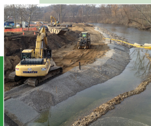
Riverfront remediation, including NAPL capping to protect the river.
