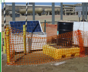
A solar powered hydrocarbon recovery system at a natural gas plant.
